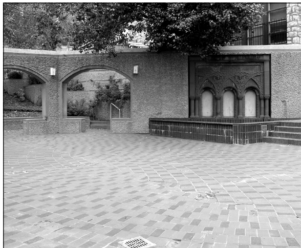
photo by Chris Morrison Water in the Diocesan Close does not drain well, which causes water to get into the Diocesan Center and Clergy Sacristy in the Cathedral during heavy rains.
